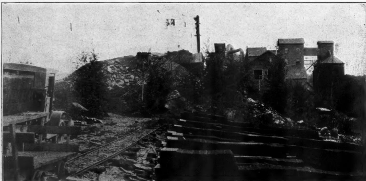
General View of Crushing Plant with Roofing Slate Storage and Tracks
